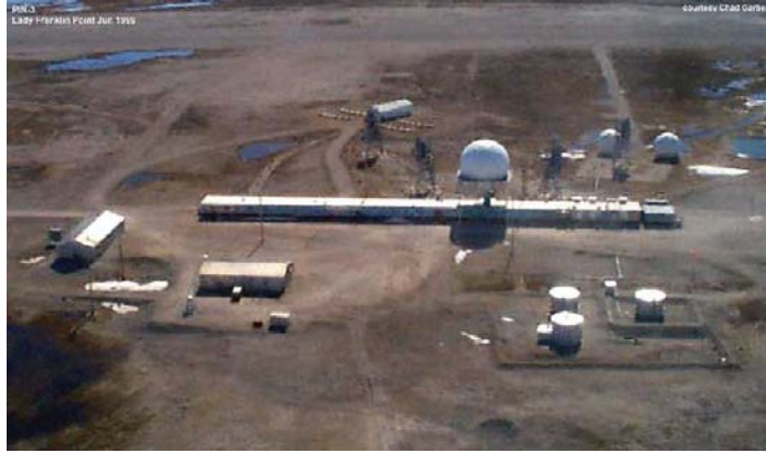
PIN-3 Lady Franklin Point Long-Range (FPS-117) Radar Site 51
