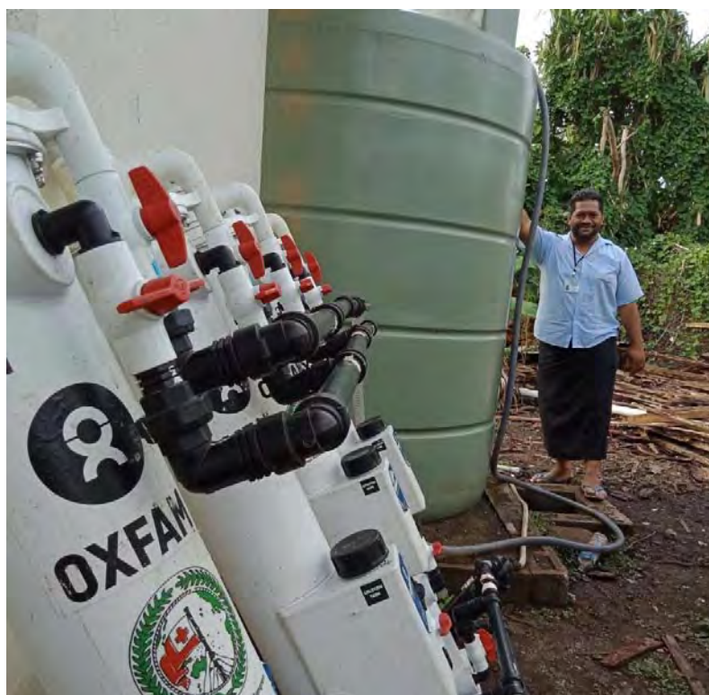
Figure 2 – Rain Water Collection and Purification System in Tonga
