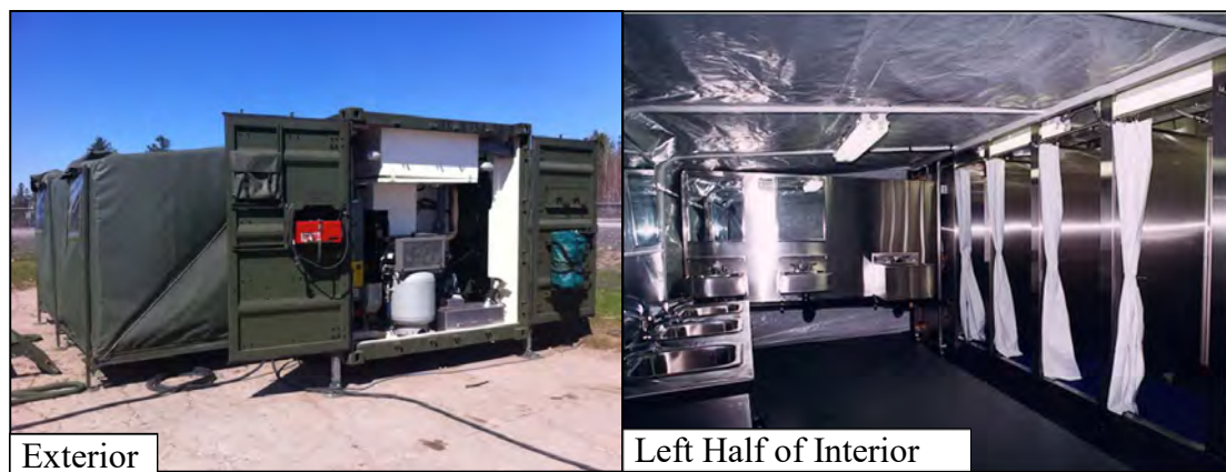
Figure 2.6 – Interior and Exterior View of Mobile Expandable Container Configuration Ablutions. 38
