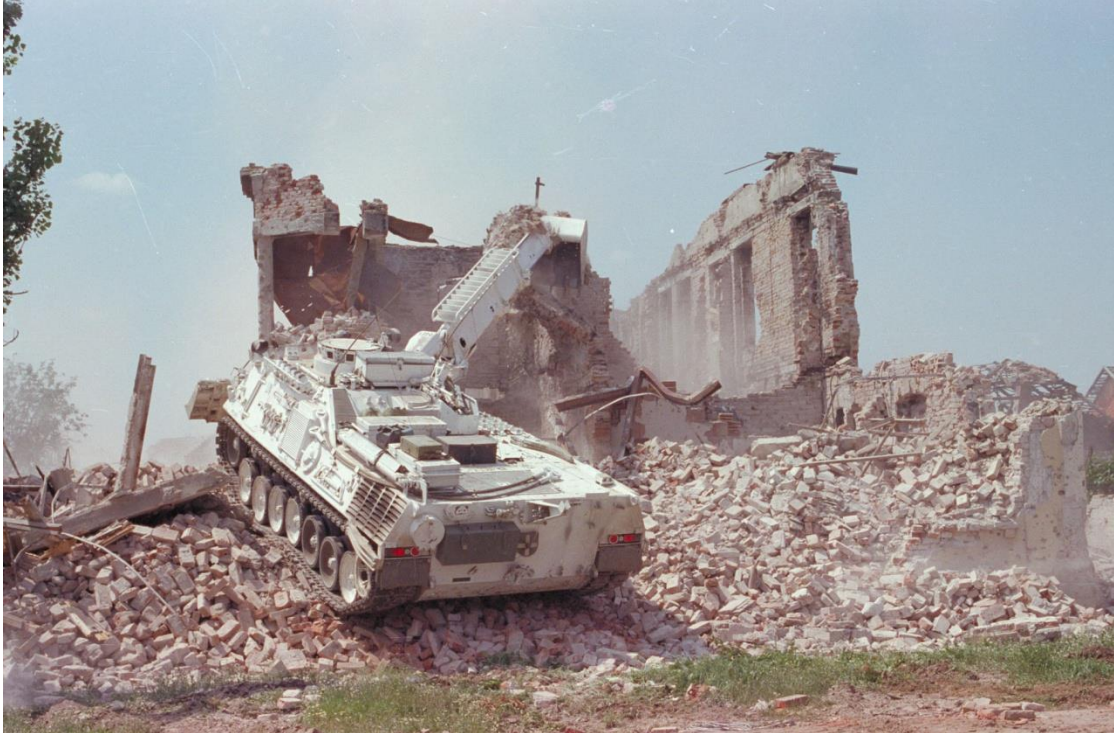
Photo XXX 143 : In May 1992, Canadian military engineers deployed on UNPROFOR use a Badger armoured engineer vehicle to demolish a damaged building Vukovar, Croatia, which is beyond repair.
