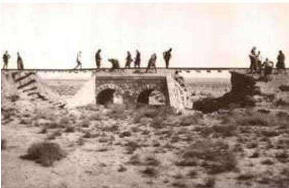
Pic.5 Turkish work party repairing demolitions to the Hejaz Railway 38
