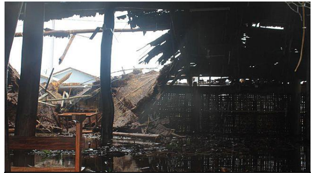
Damage left behind from Tropical Cyclone Pam in Port Vila, Vanuatu, was captured in this photo by World Vision on Saturday, March 14. Source: http://www.accuweather.com/en/weather-news/photos-deadly-tropical-cyclone/43778587
