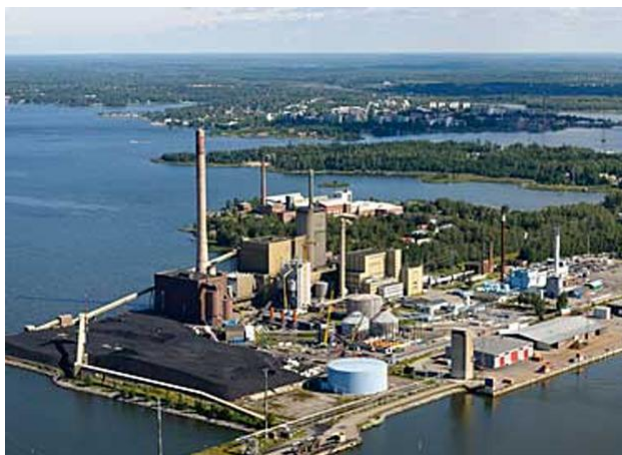
Figure 5: Biomass Energy Plant, Vaskiludon Voima Voi in Vaasa, Finland 56
