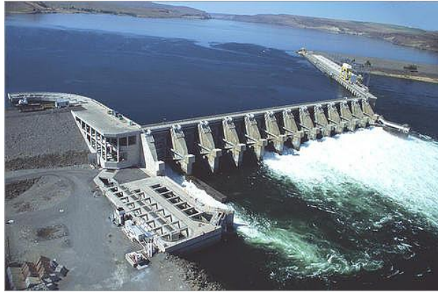
Figure 2: Priest Rapids Hydroelectric Dam, Columbia River, Washington State 38
