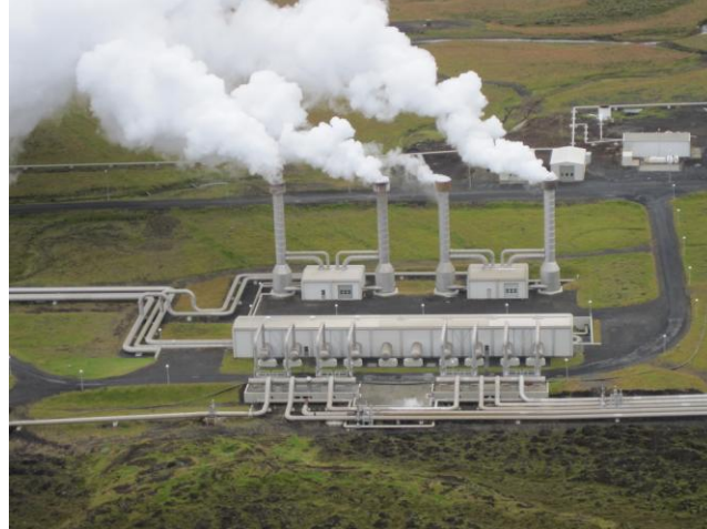
Figure 3: Nesjavellir Geothermal Power Plant, Iceland 44
